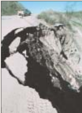
Thanks to the Small Central American Valleys (SVP) project, the Honduran government documents in the pilot valleys of the program that following Hurricane Mitch (1998), the communities lost no lives from either flooding or landslides.
